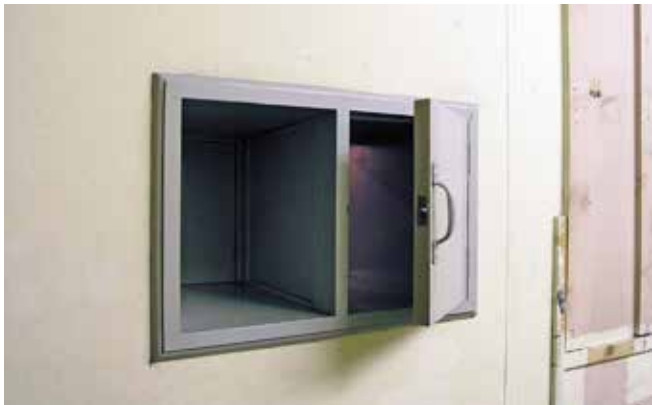
Hatchway from Message Room. Photo Victor Smith
